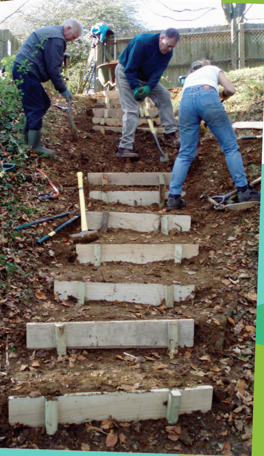
Step Installation Three Corner Copse
